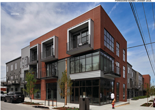
Six10 Merritt, in Nashville, Tenn., is a sub-condo within The Finery master condominium, which will continue to be developed over several years. The townhomes and flats are helping to revitalize a former industrial area and alleviate the city's housing shortage.
